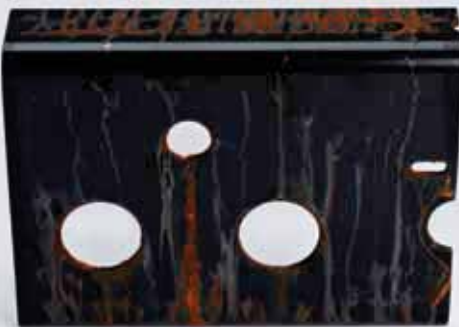
Significant rusting and blistering
