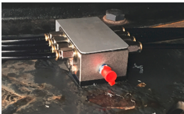
Fig.: 14 - Installation complete
