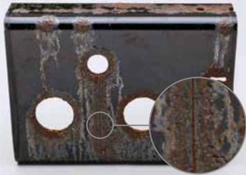
Significant rusting and blistering
